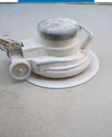
Smoothing the surface with a steel disk
