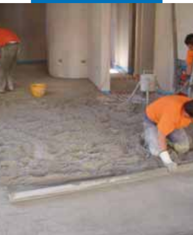
Spreading the mix with Mapescreed 704 admix
