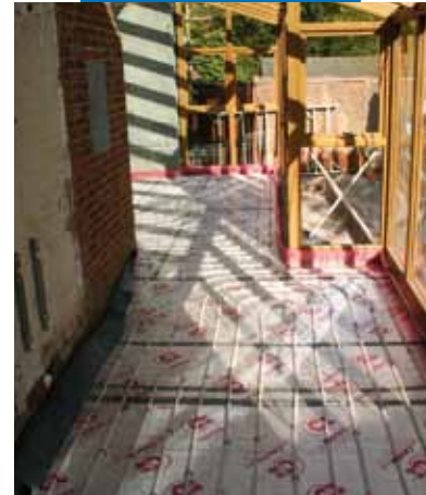
Underfloor Heating preparation
